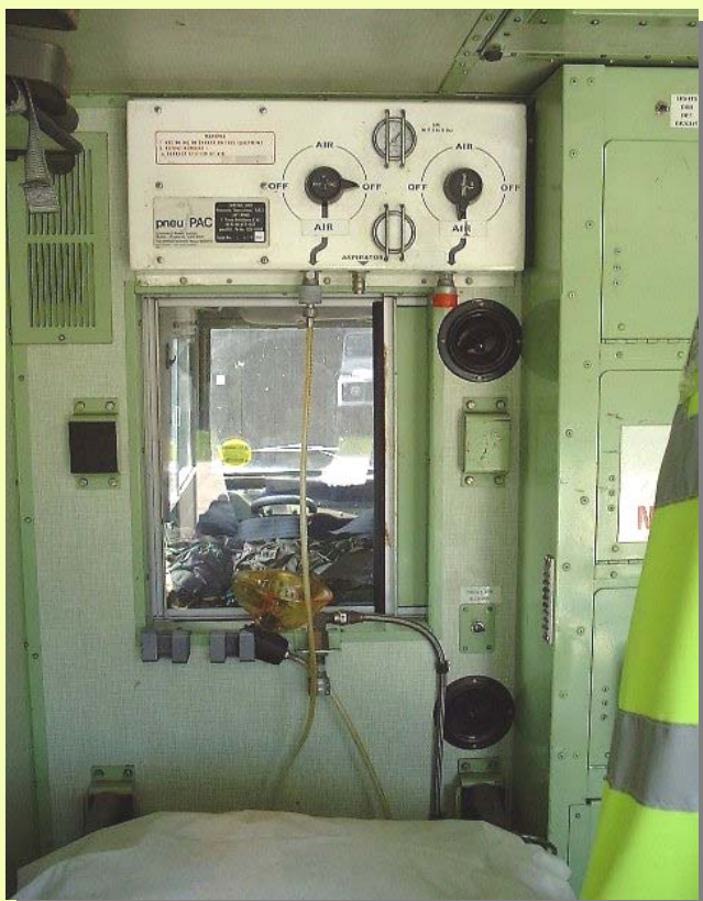
Pneu-Pac installation in 101
